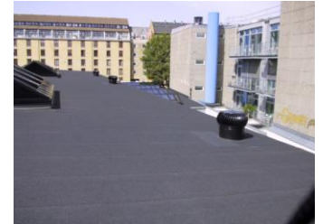
Ready to use wind turbine on a flat roof with roofing felt covering.
